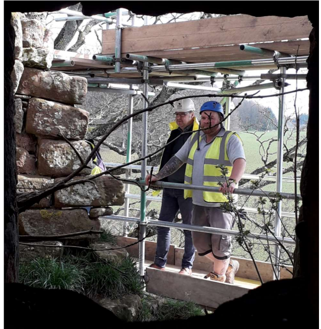
Repair of Kirkoswald Tower
