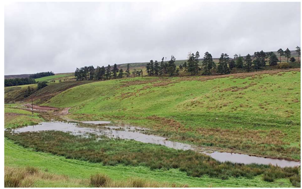
Woody dam collecting water and Sumburgh after construction
