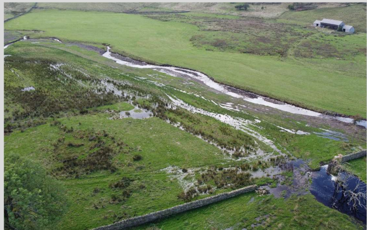
Howgill Beck ~ pre and post renaturalising work
