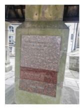
Granite: This rock formed from magma cooling and crystallising within the Earth's crust. Shap Granite, a speckled rock with large pink crystals of feldspar, has been used for decorative purposes here in Alston. It was quarried on the eastern side of the Lake District around Shap Fell and crystallised around 390 million years ago.
