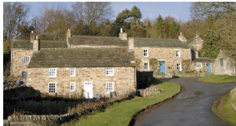
'Blanchland – use of locally worked sandstones as building and roofing stone' © B. Young, BGS, NERC
