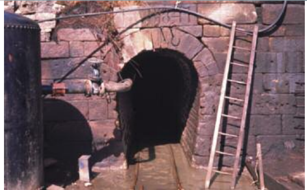
The original stone-arched entrance to Cambokeels Mine, Weardale, driven in the mid-19th Century. © B. Young, BGS, NERC
