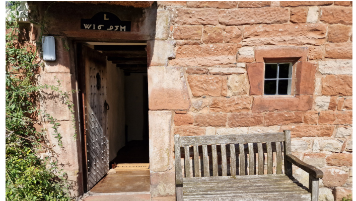
Datestone over door to the cross passage. The fire window is seen on the right. (Andrew Carter)
