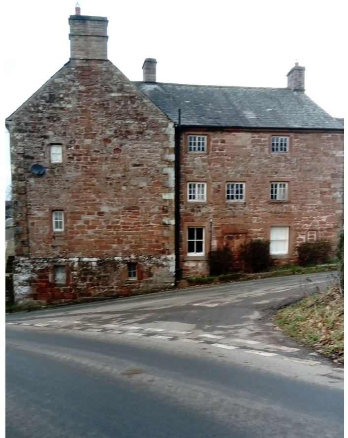
The Mansion House, older side showing earlier door (now blocked) and blocked mullioned window.
