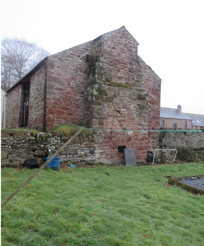
The gable viewed from the road, showing the massive external chimney stack, (an unusual feature on a bastle) and the ramp into the first floor entry to the bank barn. (Ruth Lawley).]
