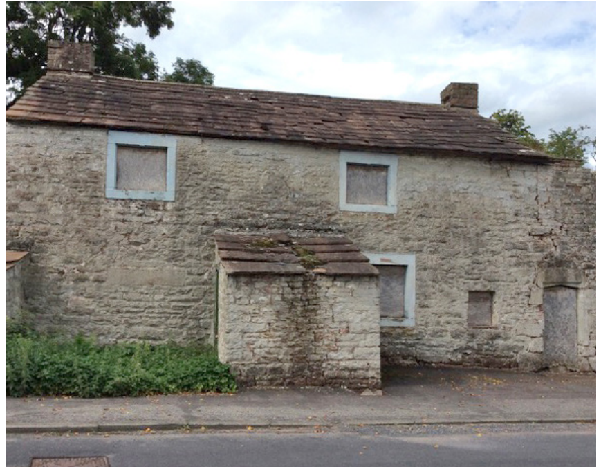
Town Foot Farm. Now derelict. Note the fire window on the right to light the inglenook of the hall or living room.
