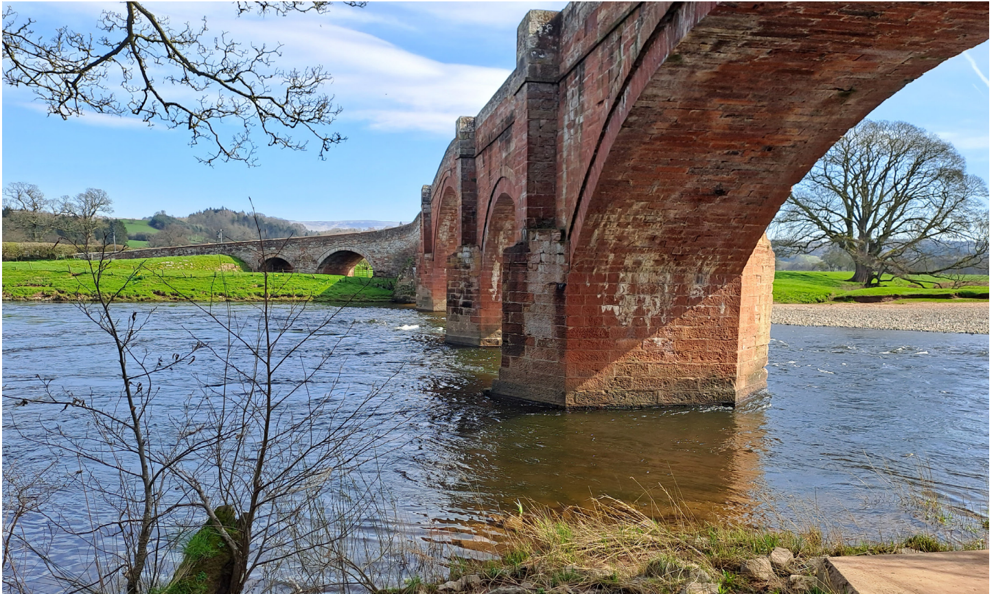
Eden Bridge, seen from the Lazonby bank. Note the narrow width of the arches and roadway above. The three-sided refuges for pedestrians stand on triangular cut-waters which allow the river water to pass smoothly through the arches. The land arches on the far bank take flood water when the river spills over the banks.
