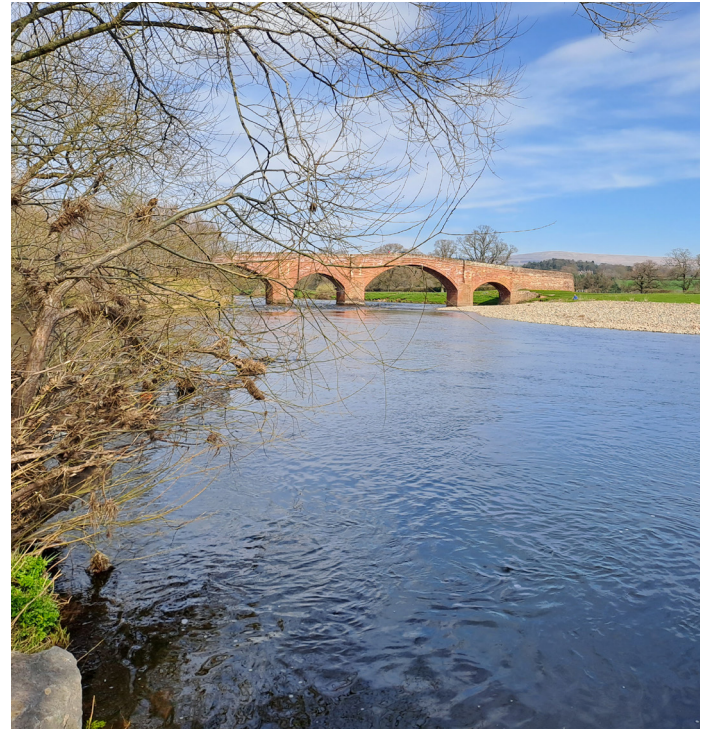
Eden Bridge. Still a major crossing on the B6413. (Roy Hill)
