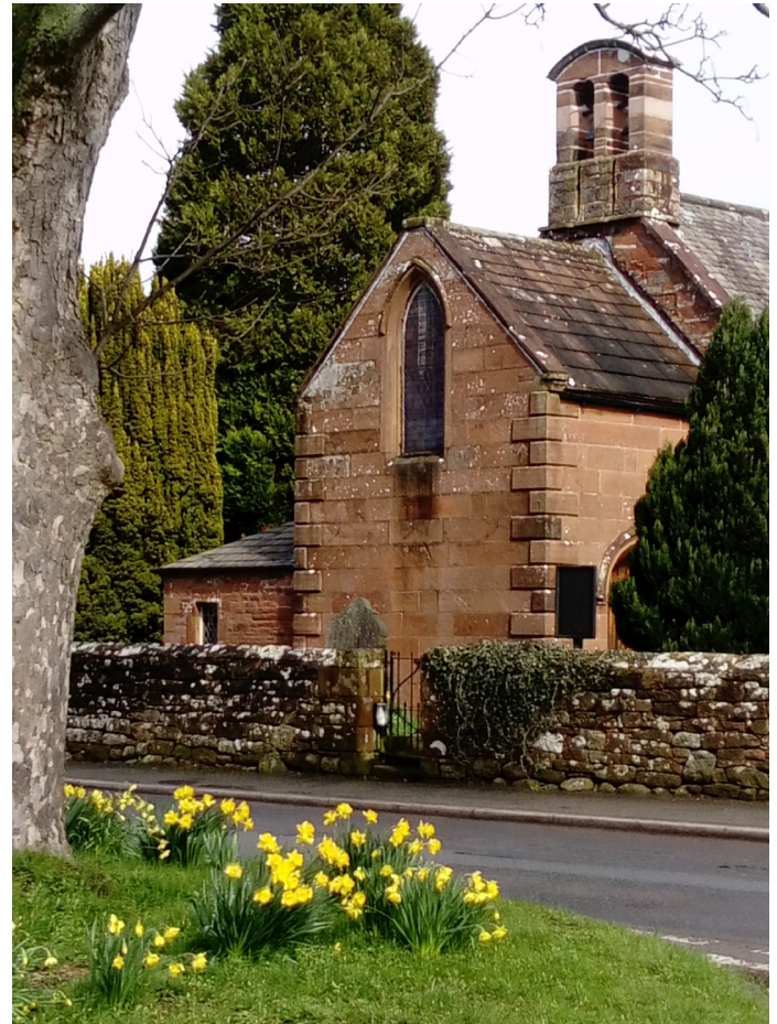
Church of St. Peter, partly rebuilt in 1718
