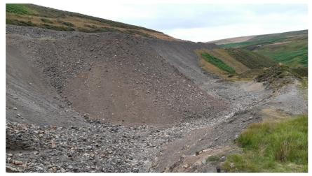
The first phase of two innovative projects to reduce metal pollution from abandoned lead and zinc mines near Middleton-in-Teesdale has recently been completed. The measures, which include building 300m of new riverbank walls and sowing an array of grass and plant species on metal-contaminated land, will limit metals being washed out of mine waste material and polluting Little Eggleshope and Great Eggleshope becks, both tributaries of the River Tees.
