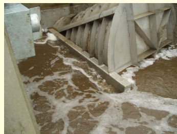
The Hydro-brake during construction
