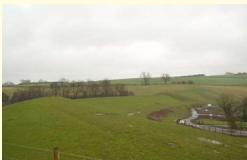
The Dam at Spring Gardens
